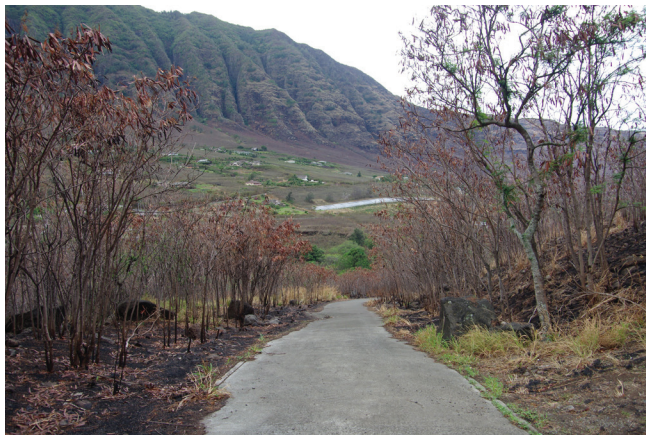
Figure 3. This access road in Makaha Valley, O’ahu, was intended to serve as a fuel break but failed due to the lack of vegetation management along the edges.
